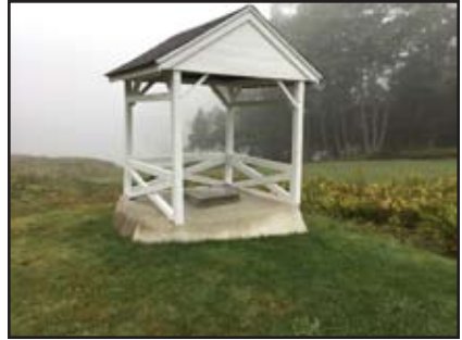
Well House, Cornelius Tarbox, Jr. House
